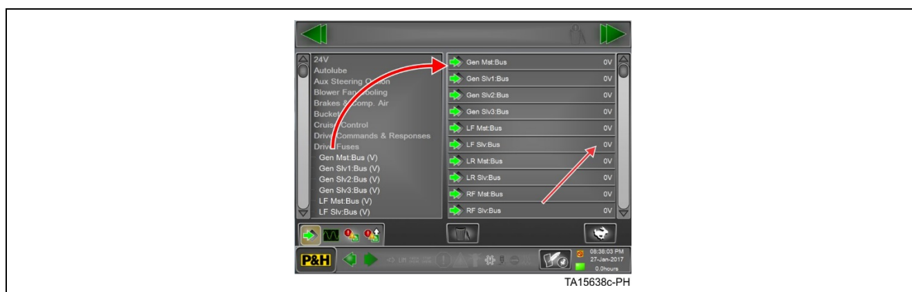
Bus voltage indication
